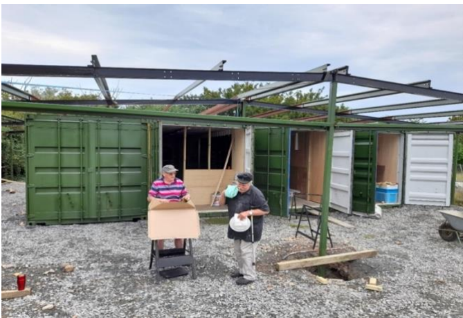
Construction of the pent roof and wings.
